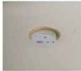
Figure: 20 Heat Detector (Picture Courtesy Wikipedia)
