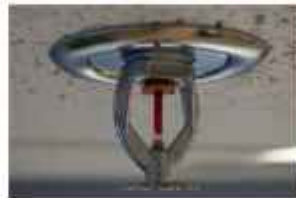
Figure: 22 Water Sprinkler (Picture Courtesy Google)
